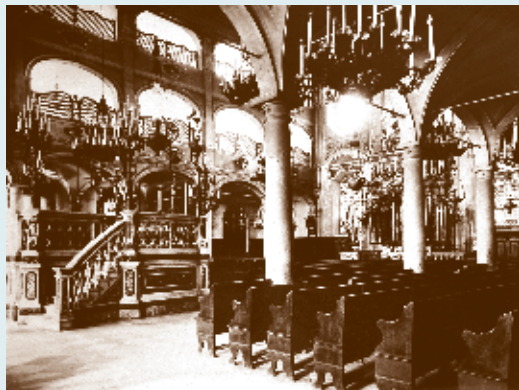
Interior of the Old Synagogue
